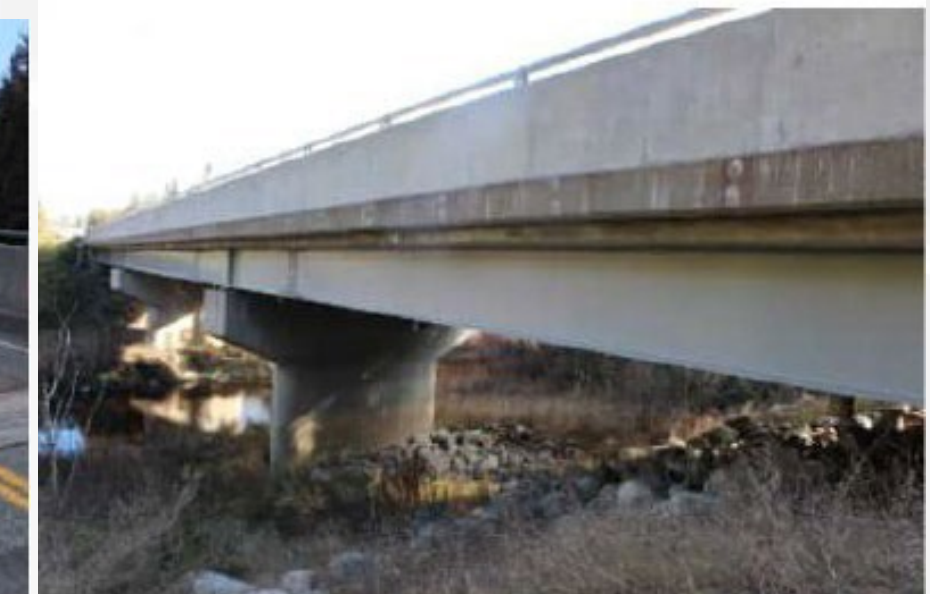
Ghost River Bridge
