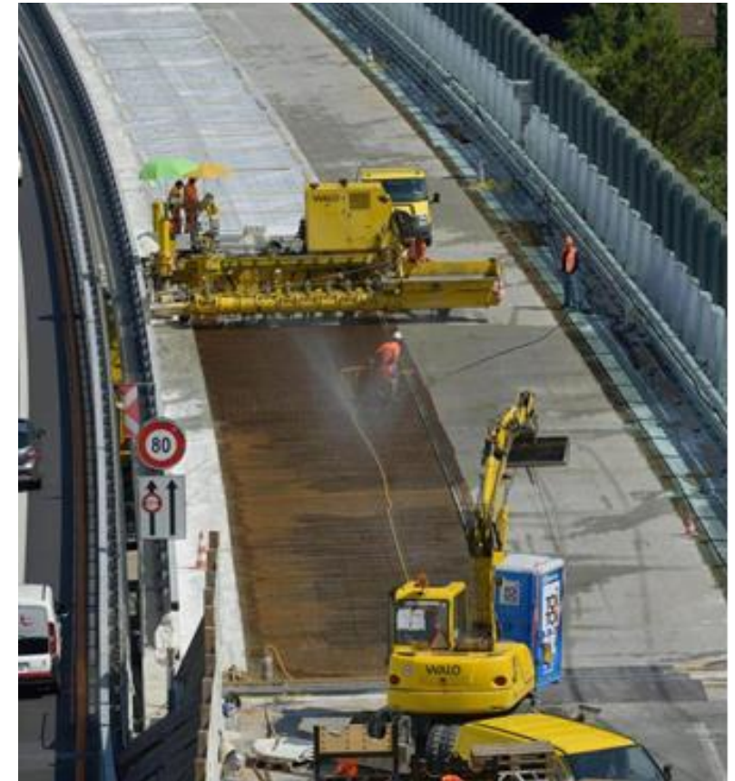
UHPFRC overlay on Chillon Viaduct near Geneva - length at 2.2 km
