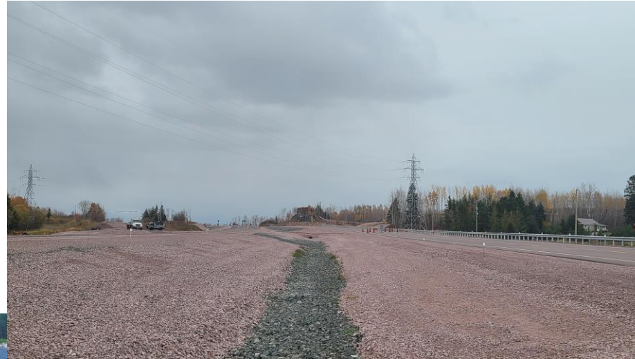
Design-Bid-Build – Highway 11/17 Expansion – Ouimet
