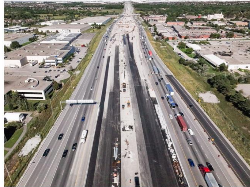
Inside lanes and shoulder paving
