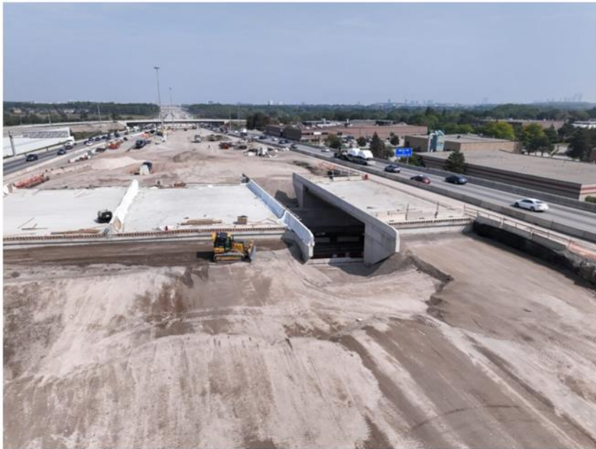
Back filling CP Rail Bridge abutment walls
